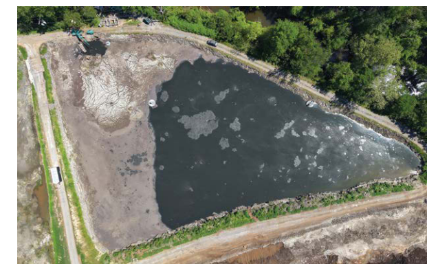
Lagoon Restoration before and after (Richmond, VA)
